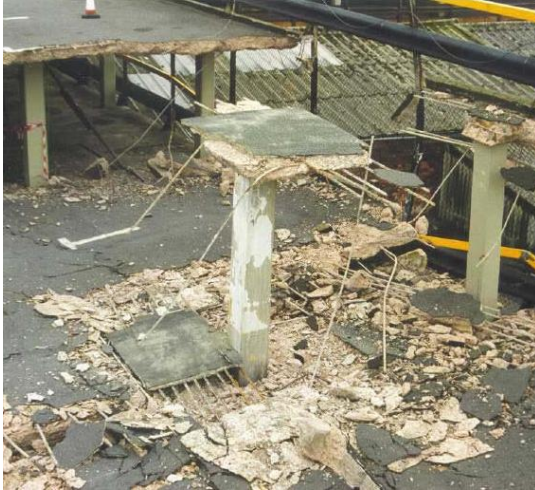
Figure 9. Typical punching shear failure (Piper's row car park, Wolverhampton, UK, 1997, built in 1965) [41]
