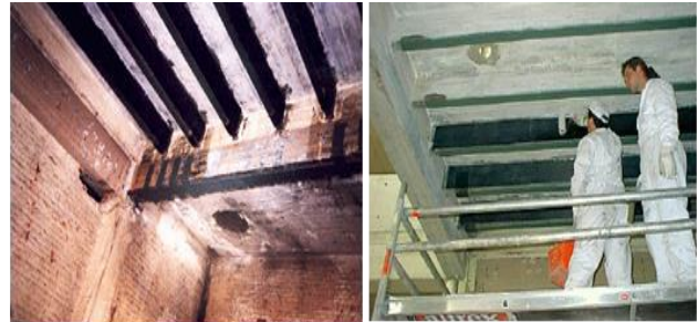
Figure 14. Hybrid strengthening of a ribbed floor slab and application of the CFRP sheets.[56]
