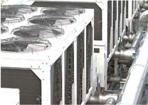
Figure 12. Solar cooling absorption chillers, [8]
