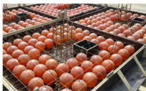
Figure 9. Fabrication of experimental bubbled slabs [40]
