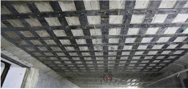
Figure 7. Steel Plate Strengthening [29]
