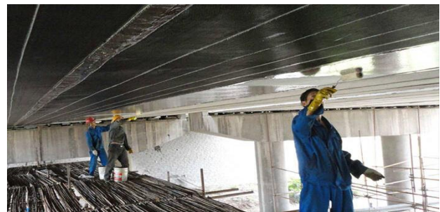
Figure 5. Strengthening with CFRP Sheets [21]
