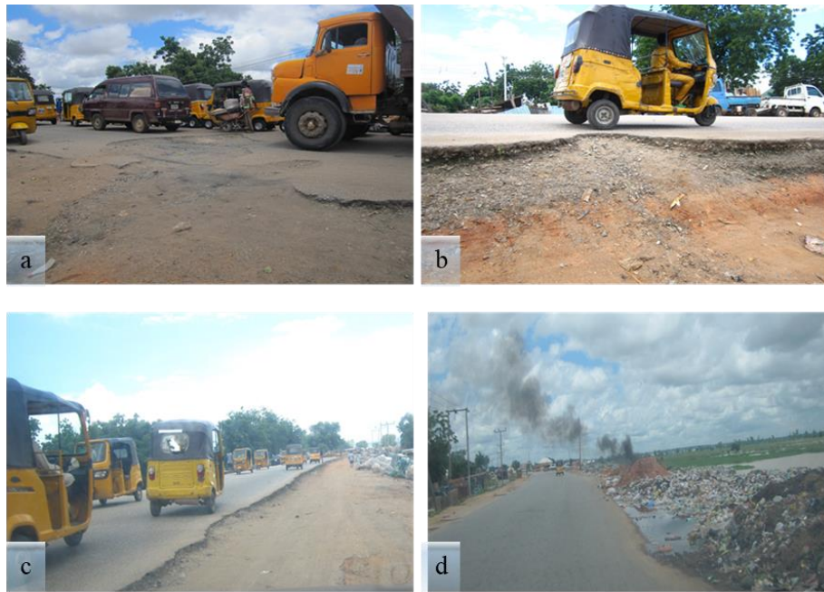
Figure 3. Physical condition survey indicating the degree of pavement section deterioration.
