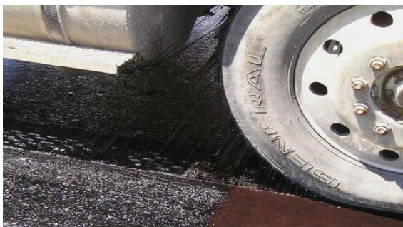
Figure 2. Tracking problem in asphalt pavement [33]
