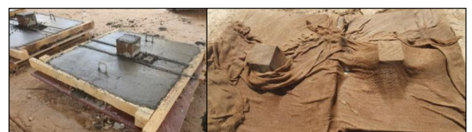
Figure 4. NC slabs casting and curing
