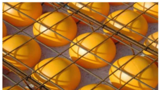
Figure13. Bubbles and Steel Arrangement
